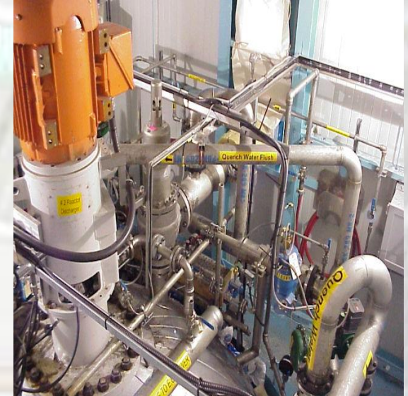
OXYGEN REACTOR INSTALLATION
