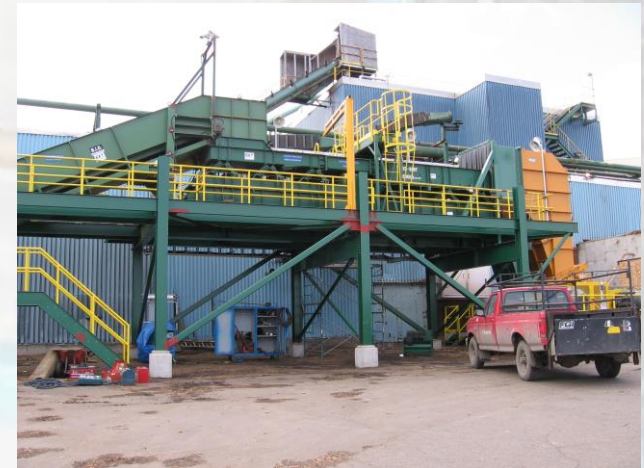
DESIGN/BUILD BOILER AND HOG FUEL UPGRADE
