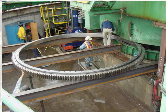
STACKER/RECLAIMER BEARING CHANGE UTILIZING 800 TON HYDRAULIC LIFT SYSTEM
