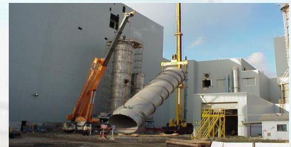
OXYGEN REACTOR INSTALLATION
