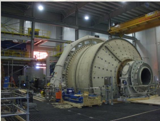
MINING EQUIPMENT INSTALLATION
